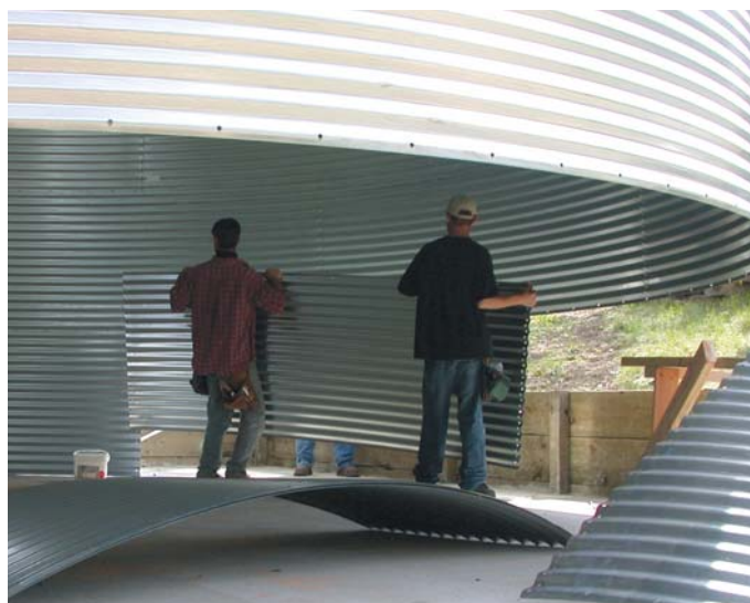
Corrugated tanks are built from the top down. As a row is completed, the tank is raised until the finished tank sits on the concrete slab, is secured, then lined with a NSF-61 potable water membrane.
