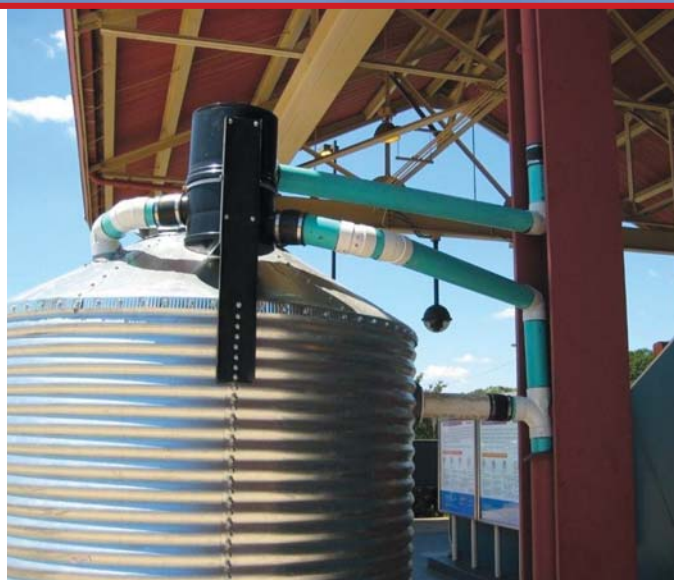
A Wisy vortex filter reduces particulate to 280 microns and is designed to handle the proper gallon per minute flow.
