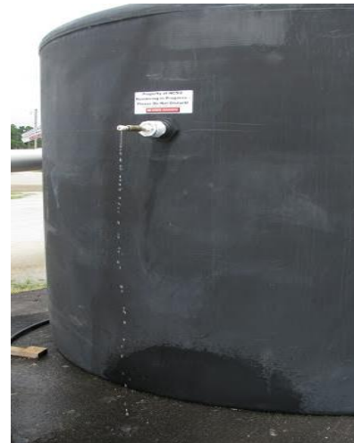
Figure 3 Rainwater Storage tank showing metered rainwater discharge available for irrigation: North Carolina State University Photo
