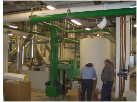
Figure 2 4.3 million gallons / year are pumped from (4) 30,000 underground tanks and filtered for use in the jail laundry
