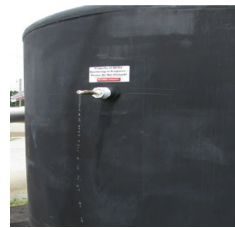
Rainwater Storage tank showing metered rainwater discharge available for irrigation: (North Carolina State University Photo)
